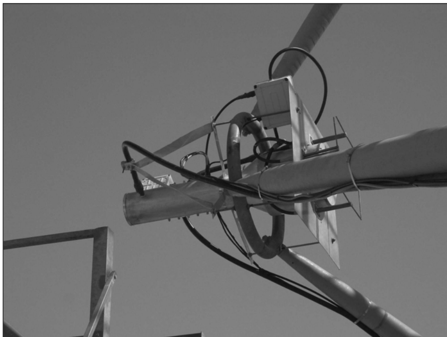
Photo 7: Feed mount in dish
